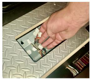
Reapply the (4) situ fixings removed in Step 2
